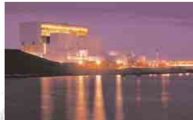
▶ Torness Power Station
