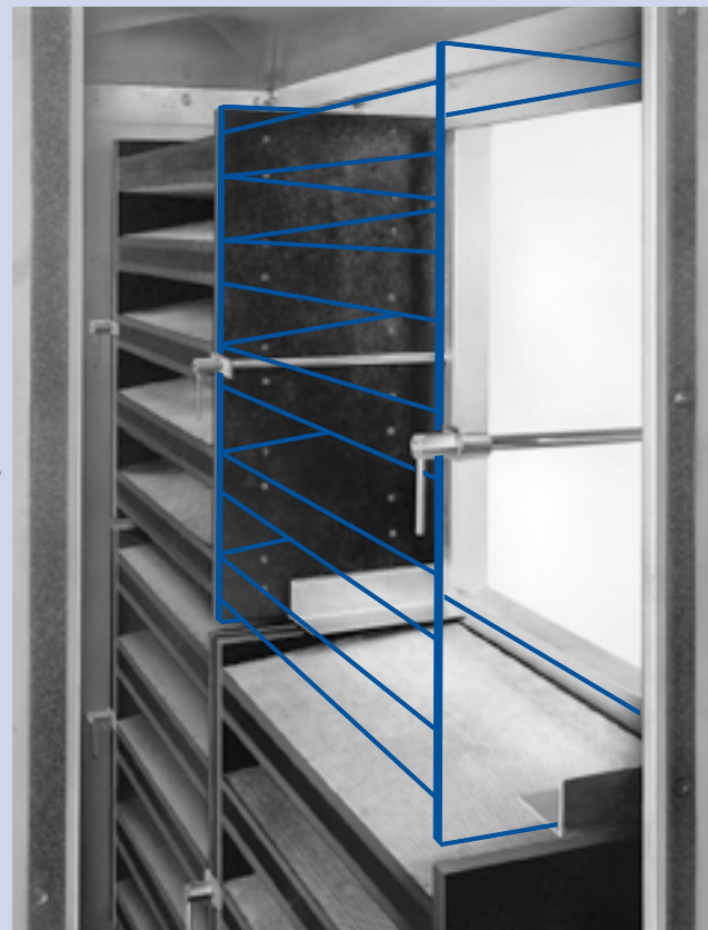
Activated carbon filter with angle supports and turnbuckle clamps
