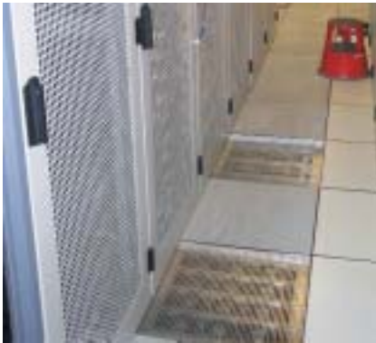
Fan Powered Computer Room Floor Grille - Cool I.T.
