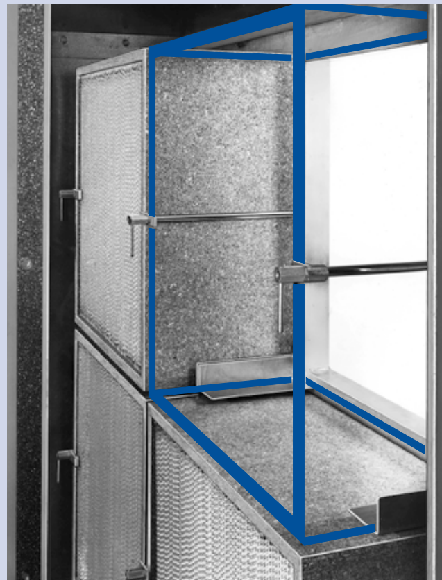
Ducted casing with support angles and thumbclamps
