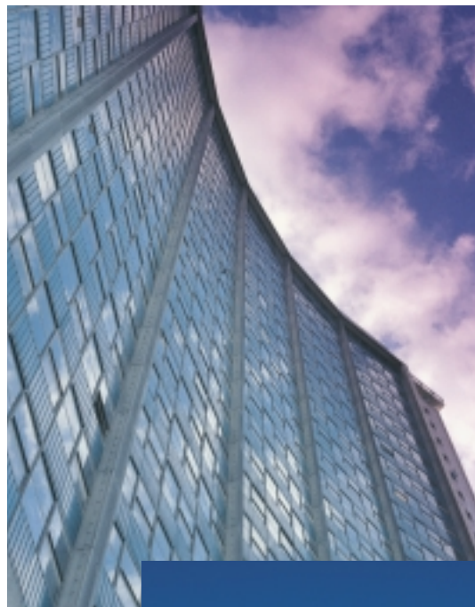
Existing Structure - circa 1960's
