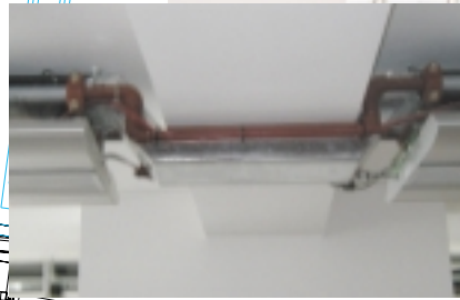
Pipework & primary duct set down
