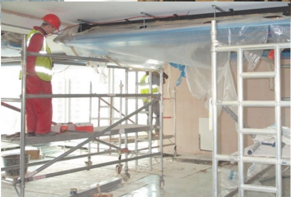
Scaffolding to access beam services
