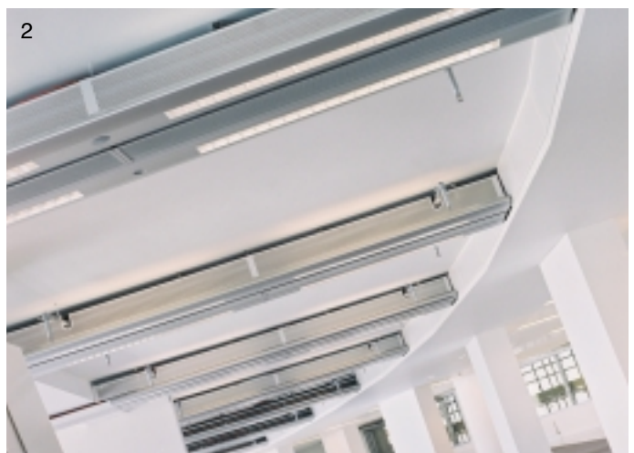
Installed flat face MSCB
